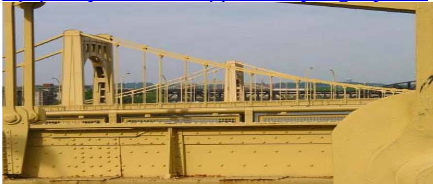
Figure 1 Towers of suspension bridge
