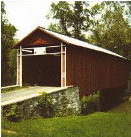
Anderson's Mill Bridge
