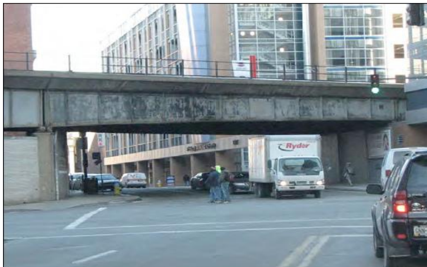
Deck Plate Girder
